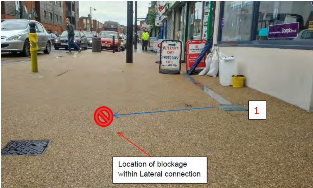
Figure 6 - Location of blockage in Desborough Road footway
