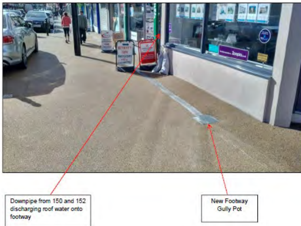
Figure 5 - New Design of footway drainage and downpipe
