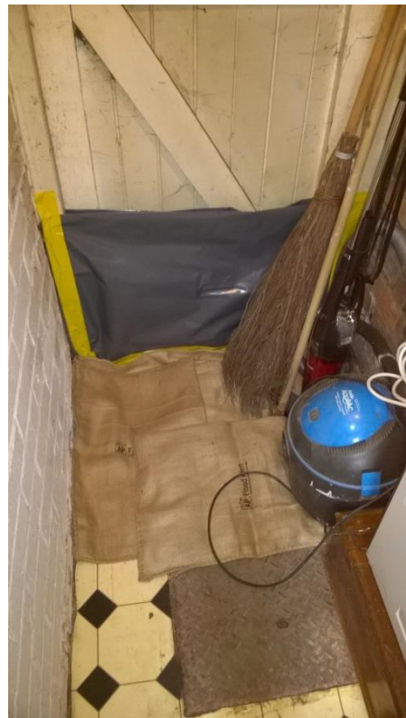
Figure F8 Back door flood protection at Arkwrights
