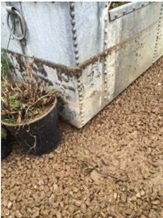
Figure F16: Flooded drive way Rignall Road to a depth of approximately 40 cm May 2018
