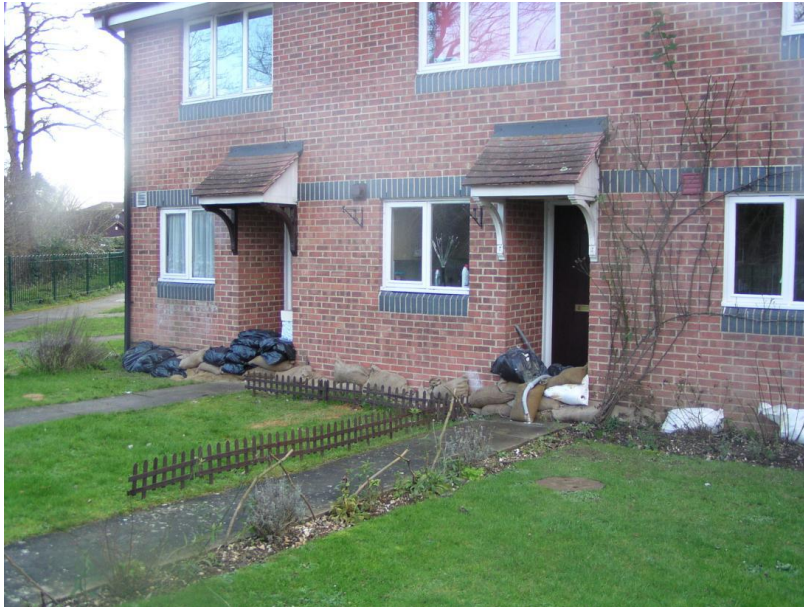
P1010131 TQ0497585128 looking SW 43-42 Oakside Significant sandbagging, though no riverside flooding reported.
