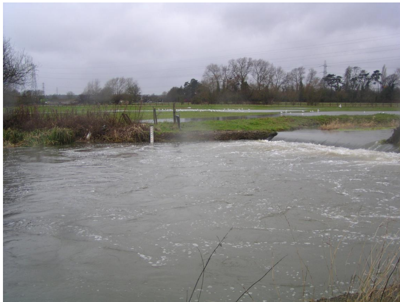
P1010114 TQ0518685568 Looking W g-b location
