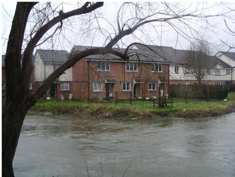
P1010108 TQ0500185118 Looking W to Oakeside Evidence of sandbagging in Oakeside properties, number 42-44, from Willowbank Island.
