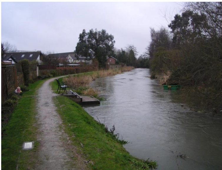
P1010099 TQ0501385015 Looking S d-s Rebuilt flood defence between Poplar Road and Alder Road. Maximum water level reported by residents as to just below the middle step of the fishing platform.
