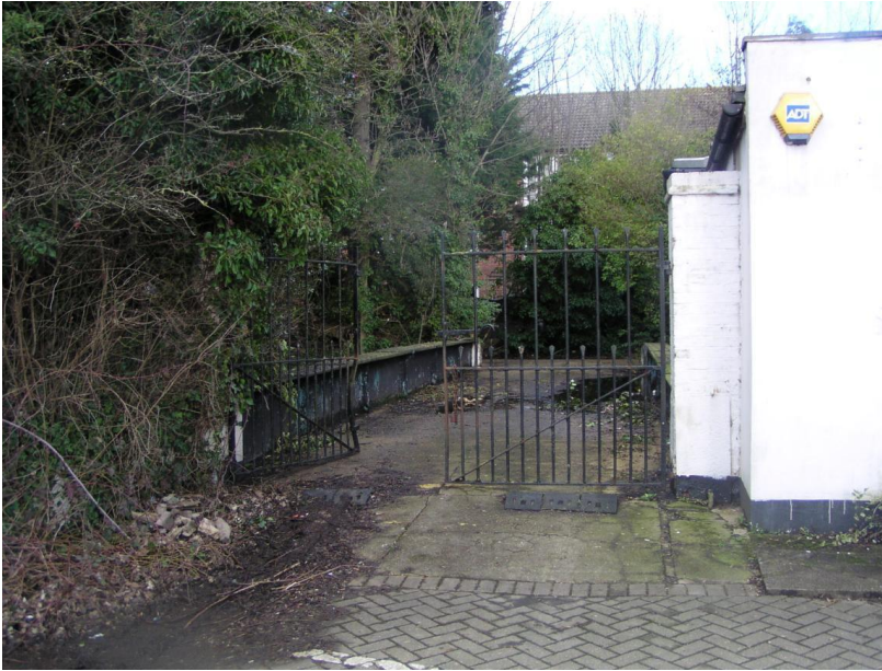
P1010148 TQ0500184790 Looking NE Bridge
