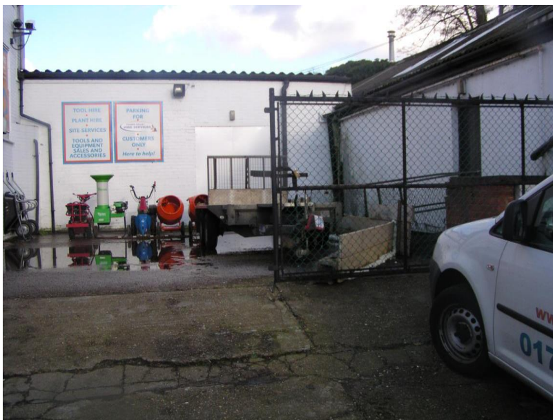
P1010149 TQ0502684761 Looking NE TV Hire Temp defence Thames Valley Hire Services entrance and temporary defence (scaffold boards and foam sealant to the right).
