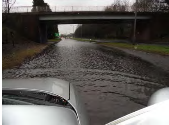
Road flooding, A413. Photo courtesy of CSP Parish Council, February 2014
