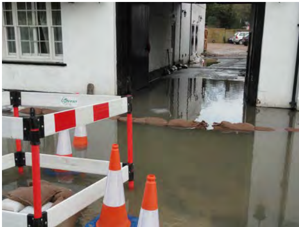
Flooded entrance to the George Inn. Photo courtesy of CSP Parish Council, February 2014
