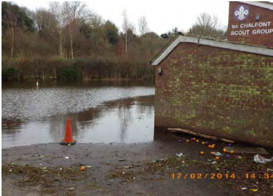
Flooding outside of the scout hut. Photo courtesy of EA, 14/02/17
