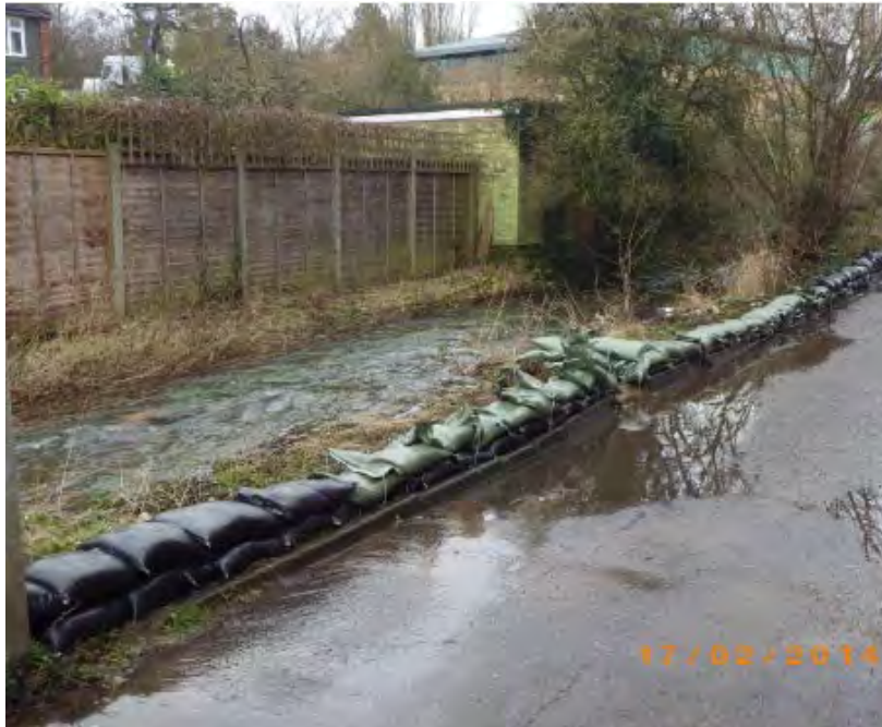
EA sandbag wall protecting industrial area and Hiljon Crescent. Photo courtesy of EA, 14/02/17
