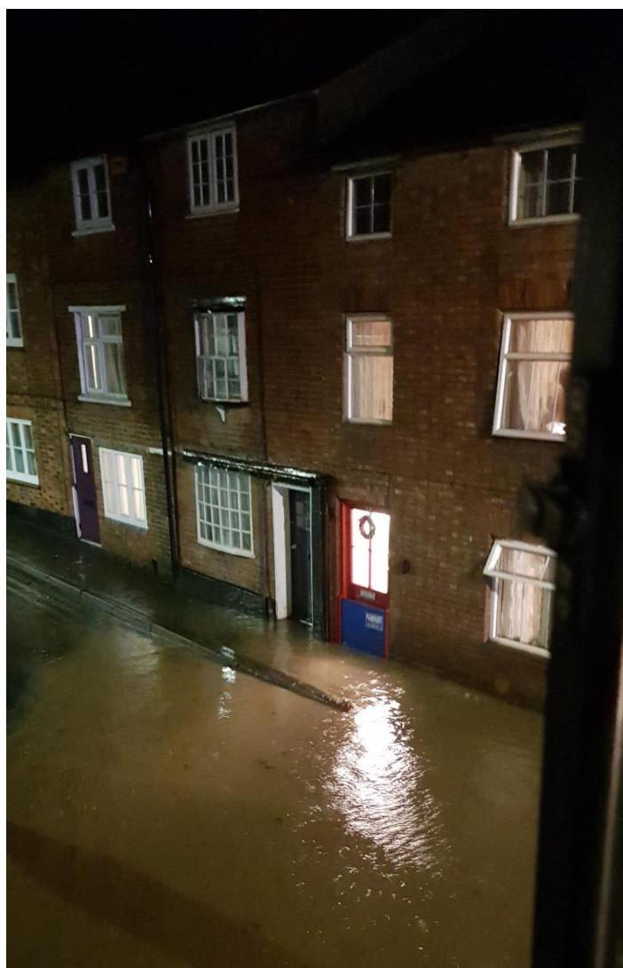
Figure 7-1: PFR deployed at Nelson Street, 23 December 2020 (photo credit: Sharon Oaks)
