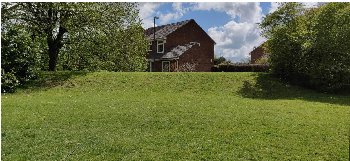
Figure 5-3: Flood defence embankment at March Edge, Linden Village
